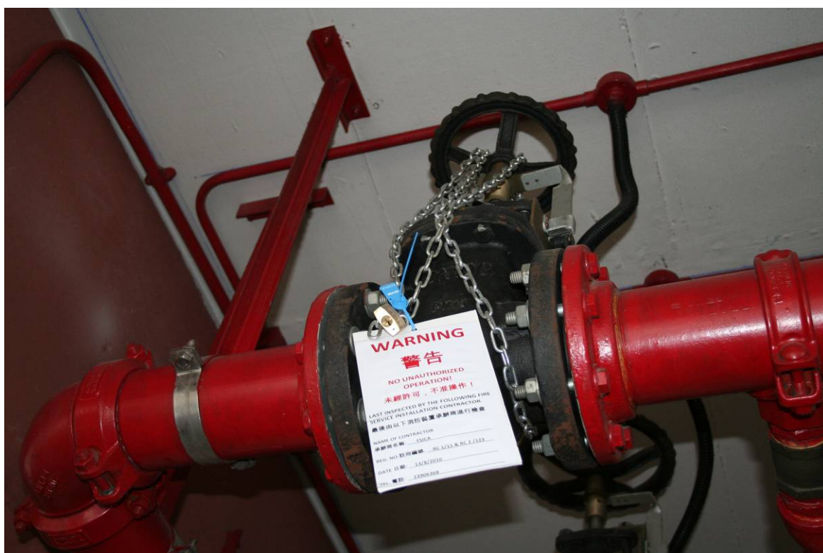
Typical Method of Securing the SSSV
