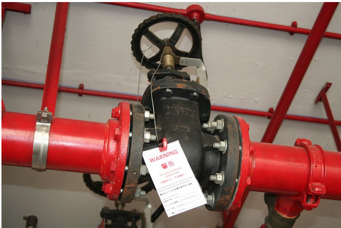
Typical Method of Securing the SSSV
