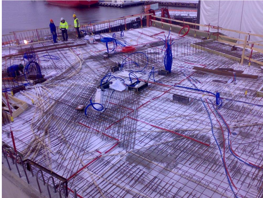
Example of a construction site using the MLC-S piping
